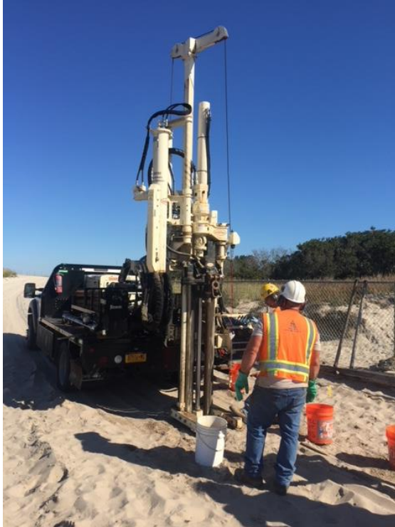
Figure 8. Geoprobe sampling at Robert Moses State Park, Oct. 2017.
