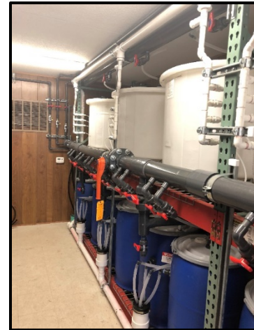
Close-up of Experiment Columns
