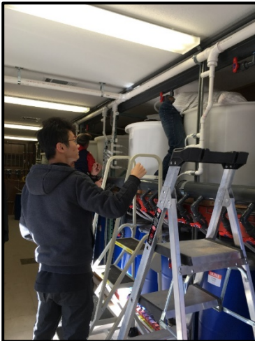
Staff Installing Media into Sand Filters
