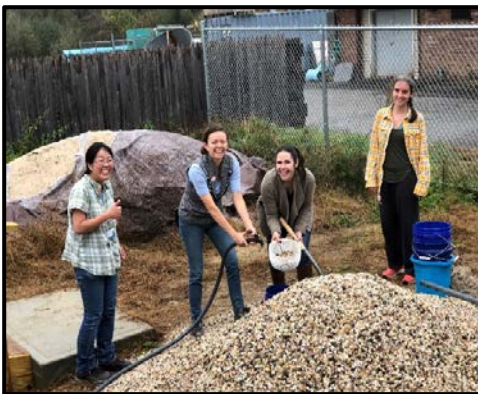
Staff Washing Gravel for Sand Filter Columns
