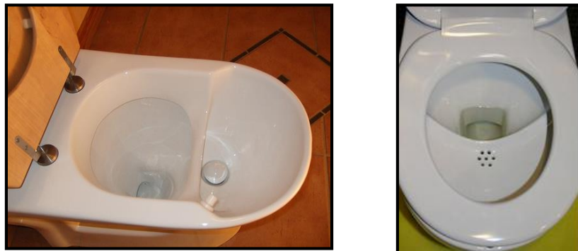
Figure 3-8: Two Swedish urine separating toilets (EcoSan and Novaquatis)
